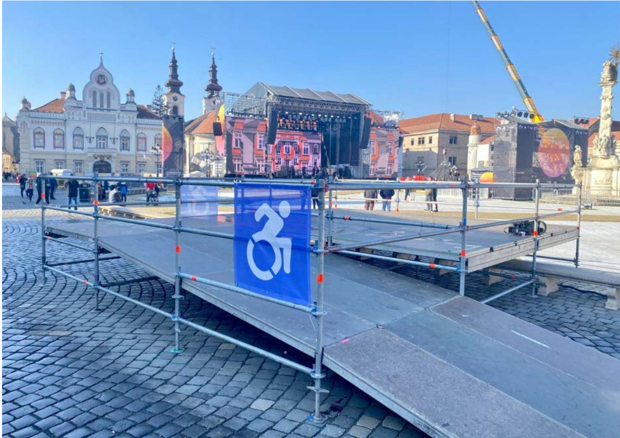
Platform with ramp for disabled people installed for the concert in Union Square | Photo: The Center for Projects
